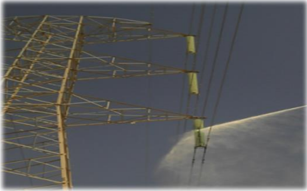
Live line washing to remove the accumulation of dirt, dust, or other materials on periodic frequency.
